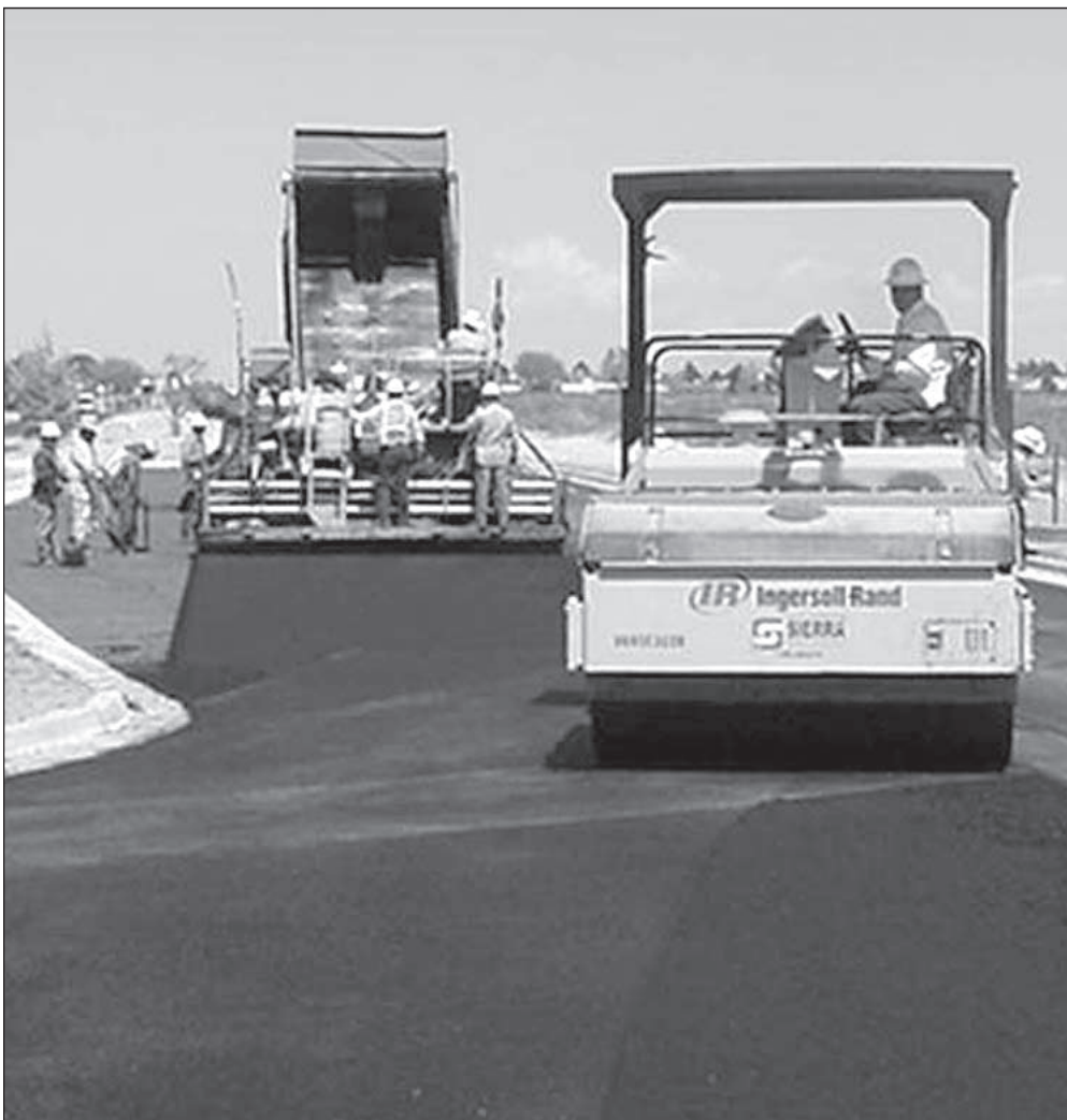
BLACKTOP — Road crews spread asphalt and rolled it smooth last week during the final stages of a street project in Horizon City begun in August 2003. The project widened all of Darrington Rd., through town, to four lanes and resurfaced all existing two and four lane portions. Coby Nichols, a TXDOT inspector, said he thought the intersection at Horizon Blvd. could be fully functional around mid-April.
