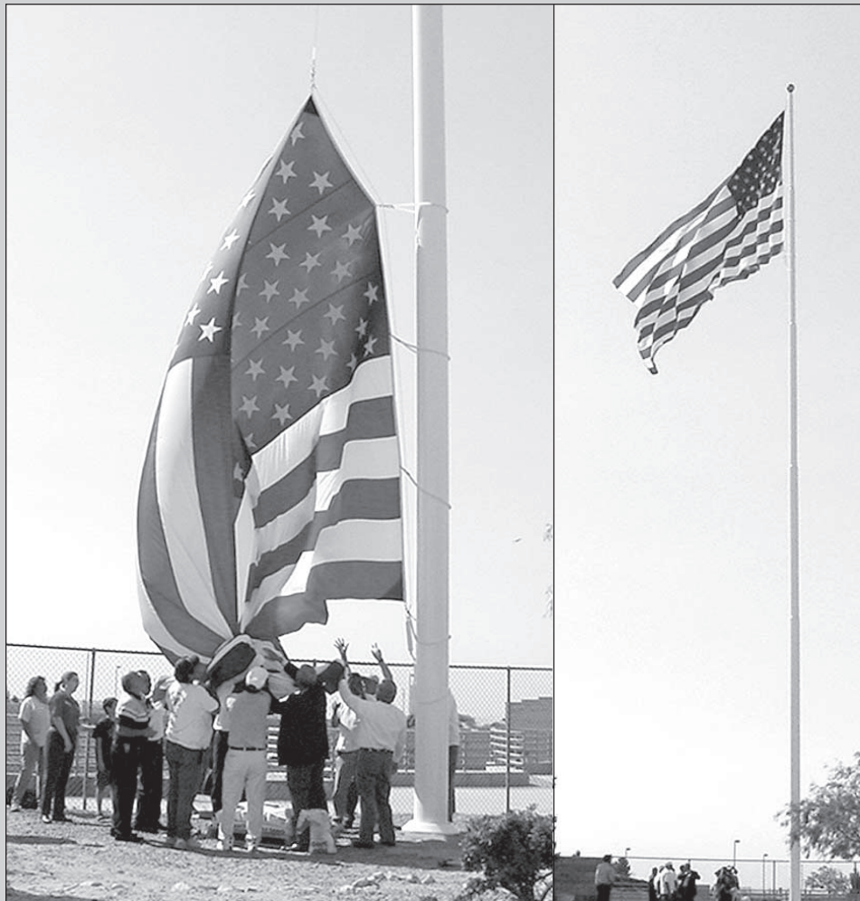
SISD WELCOMES NEW FLAGPOLE — Construction crews from U.S. Flag and Flagpole of Beaumont, Texas installed Socorro ISD's new Freedom Flag pole July 8 on the landscaped northwest grounds of the Student Activities Complex, 1300 Joe Battle Boulevard. The white, 100-foot pole, delivered in sections, was anchored and assembled July 7 and 8. The installation has been designed to support a garrison-sized flag 20 feet tall by 38 feet wide — and the District is working on plans to illuminate the flag and pole. During the past two years, community individuals and businesses donated money for the project. A dedication ceremony is being planned for this fall.
