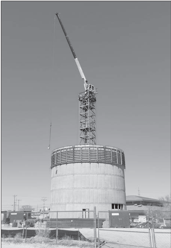
GOING UP – After the initial dirt work and gound infrastructure was in place, the construction of the elevated storage tank took off quickly. The first photo, top left was taken on February 17. The building in the background is the office for Horizon Regional Municipal Utility District 3. The bottom right photo was taken on May 27. Priming on the tank has begun, with lifting to begin shortly.
