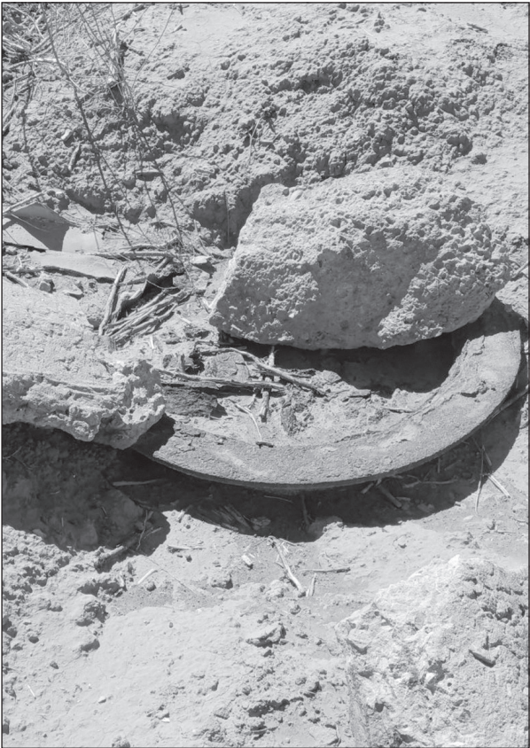
MAKE SHIFT – This LVWD manhole located behind Bovee Road is secured simply with a barrel lid and rocks placed on top of it.
